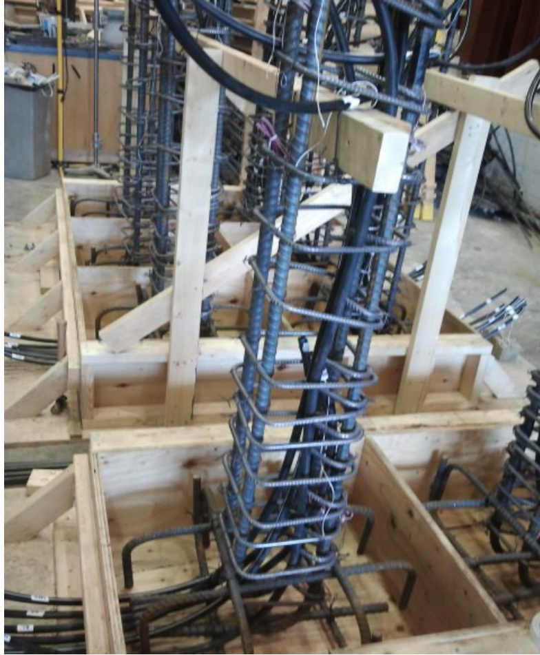
Figure 3-17: Column footing formwork with cages placed inside
