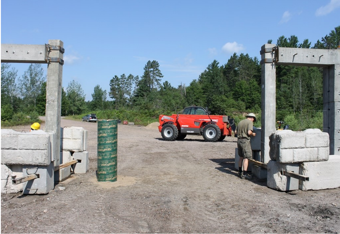
Figure 4-40: Pre-test setup of test 4 (CONV-1 and SEIS-13)
