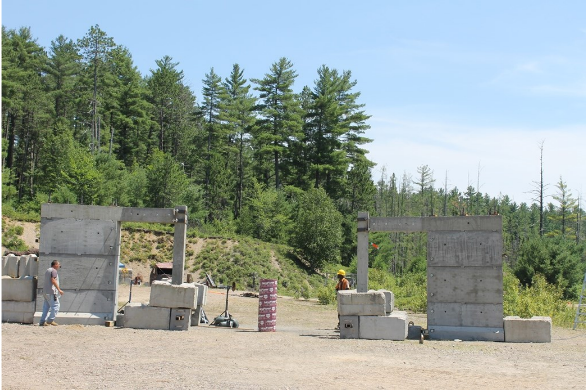
Figure 4-18: Pre-test setup of Test 2 (SEIS-9 and CONV-20)
