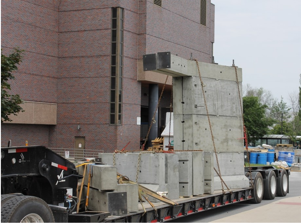
Figure 3-7: Transport of support structure to site
