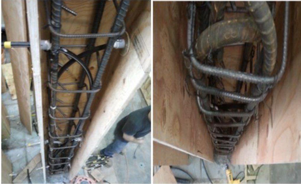
Figure 3-18: Column formwork placed around reinforcement cage
