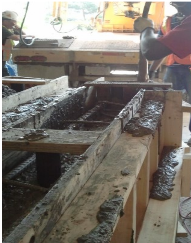
Figure 3-6: vibration of support structure concrete during casting
