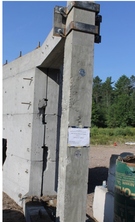
Figure 4-26: Photograph of column CONV-20 prior to test
