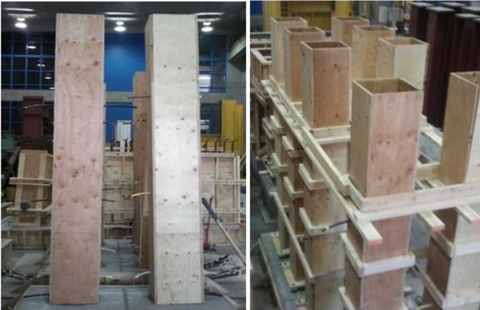
Figure 3-19: A photograph showing (a. Columns formwork and b. columns braced with 38×89 mm wood studs)
