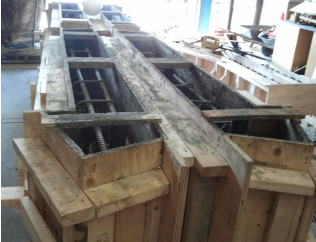
Figure 3-5: Components of support structure's formwork
