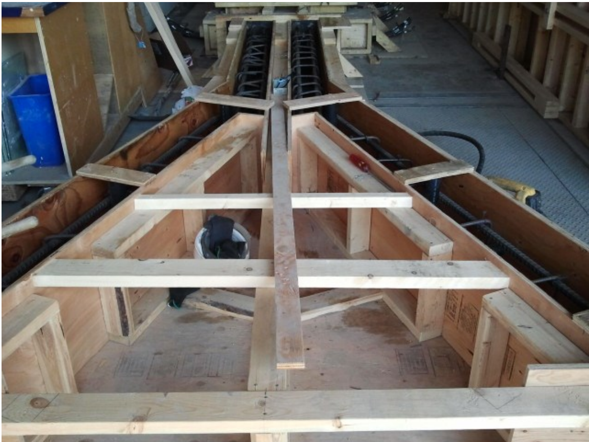
Figure 3-4: Formwork of support structure’s cantilevered Y-section
