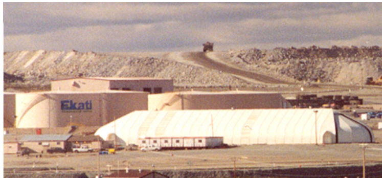
Figure 7.7 – Ekati Diamond Mine 88' x 320' Storage Facility
