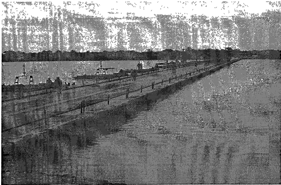
Figure 3.4 Floating bridge simply supported at shores and resting on water along its span (army-technology.com).
