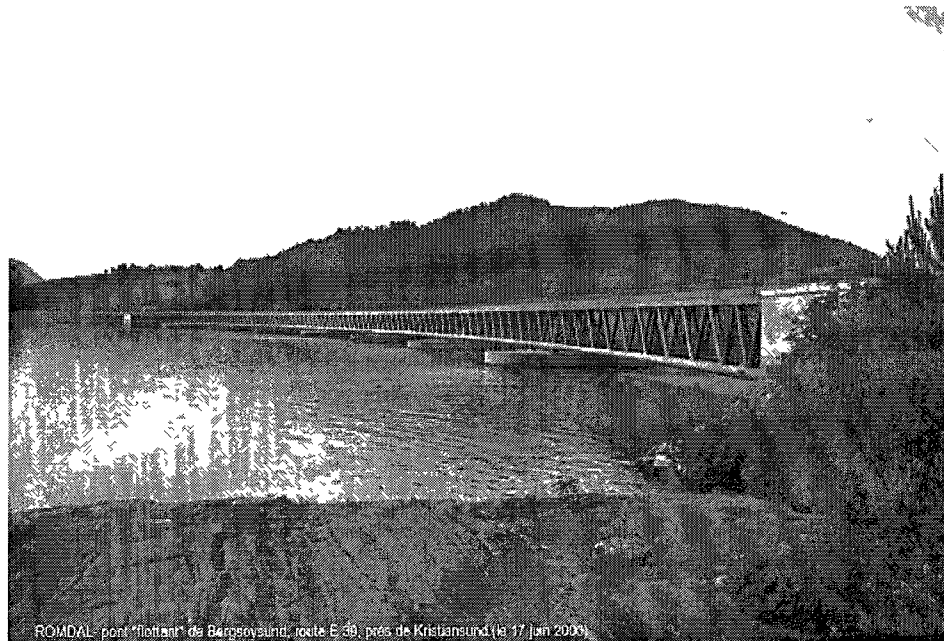
Figure 1.2 Bergsoysund pontoon bridge, Norway (Watanabe 2003)
