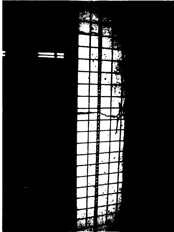
Figure 4-81: Crack Pattern After Test DB-20M-1-2
