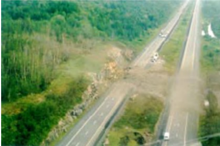
Figure 118: Aerial photograph of the accident site (Mainiero et al, 2009)
