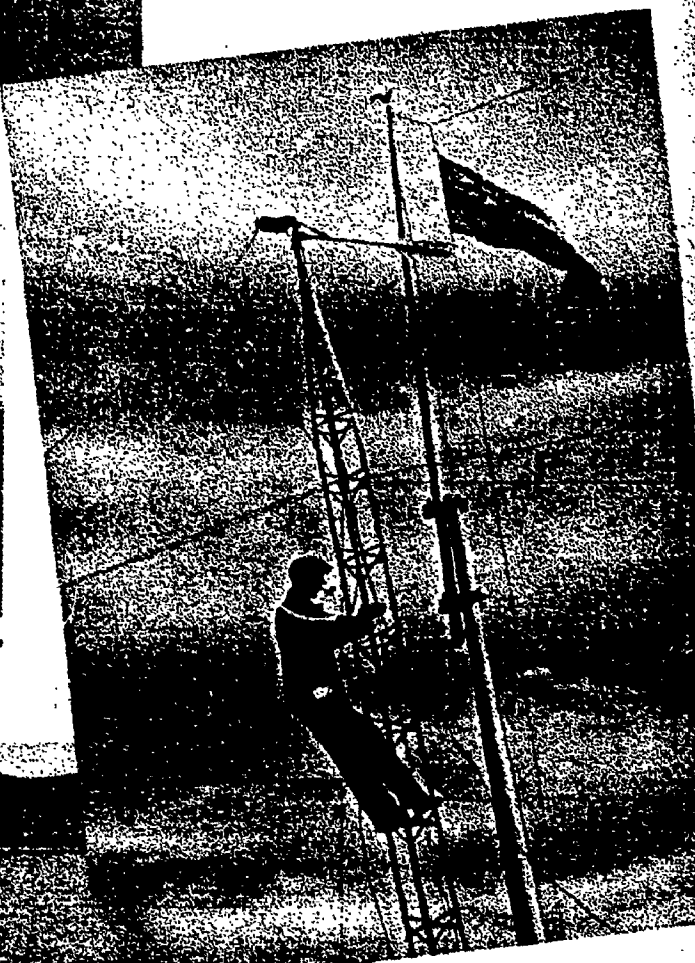
Ship's Carpenter Clem James, erecting a wind mill to charge the batteries of the radio station at Hebron.
