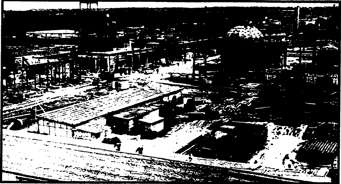
Figure 1.2 The Polymer plant under construction in early 1943
