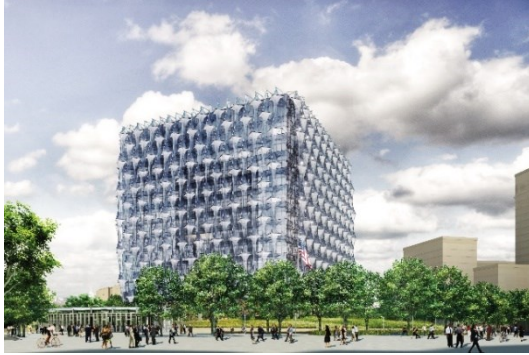
Figure 2.9: (left) artist's concept of ETFE PV double skin façade; (right) detail showing connection with inner glazed surface
