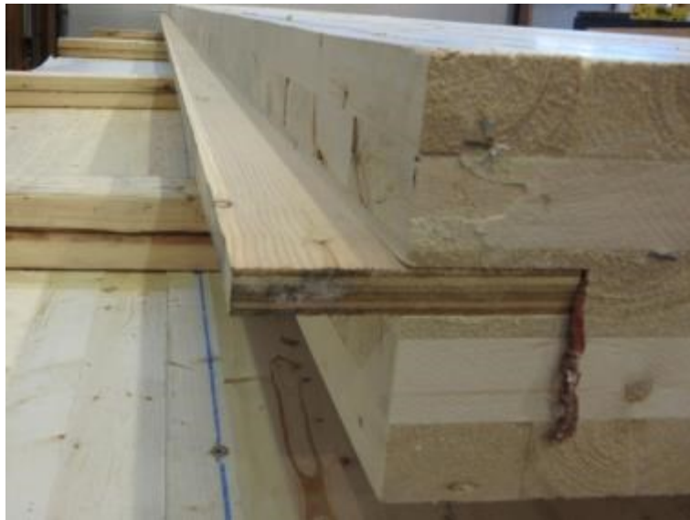
Figure 2.13 – Internal spline made from a plywood strip
