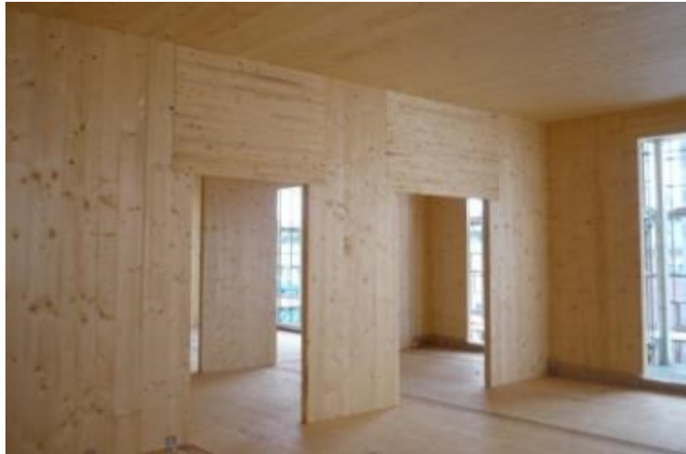
Figure 2.1 – CLT construction
