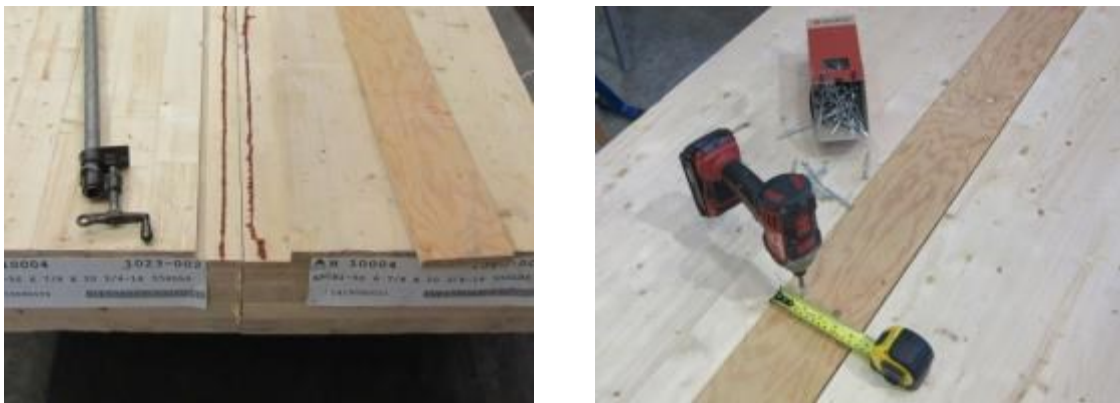
Figure 2.17 – Single surface spline made from a plywood strip
