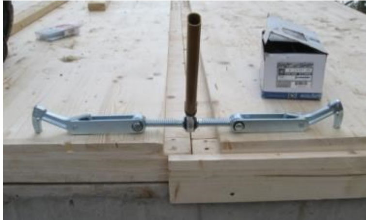
Figure 2.7 – Ratchet and hooks used for CLT panel-to-panel connection (photo: FPIinnovations)
