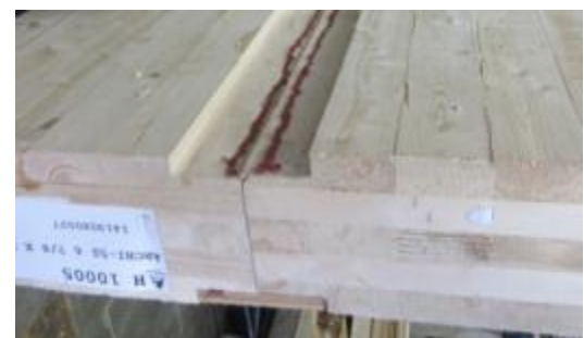
d) Double surface spline
